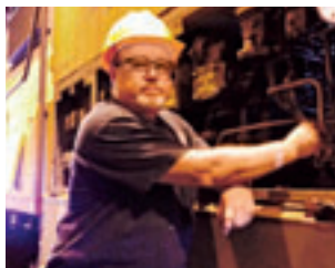
Local 334 member Randy Swanson and the piping for a positive train control modification.
