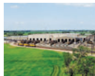
The diesel shop repair facility at Bailey Yard.
